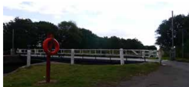
Salmonpool swing bridge
