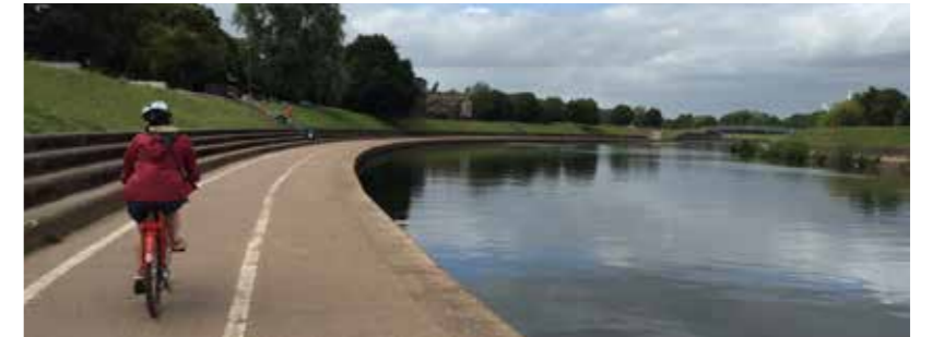
South bank of Flood Relief Channel and River Exe
